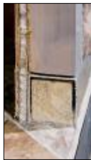
All aluminum sills and wall studs are mechanically joined and the aluminum sill tubing is fully reinforced internally with wood, providing greater strength and stability when it is "bolted-through", never screwed, to the sub-floor structure and the steel frame below.
