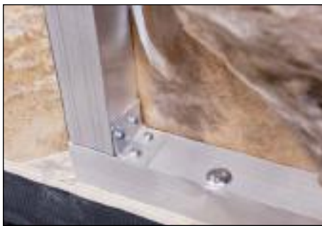
All aluminum sills and wall studs are mechanically joined and the aluminum sill tubing is fully reinforced internally with wood, providing greater strength and stability when it is "bolted-through", never screwed, to the sub-floor structure and the steel frame below.
