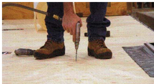
5/8" TONGUE AND GROOVE, MARINE GRADE PLYWOOD FLOOR
