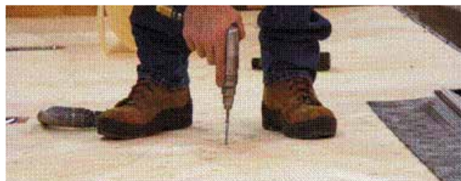
5/8" TONGUE AND GROOVE, MARINE GRADE PLYWOOD FLOOR
