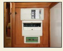
PROTECTION THE FULL BANK OF BREAKERS AND FUSES FOR INTERIOR COMPONENTS ARE CENTRALIZED FOR QUICK REPLACEMENT
