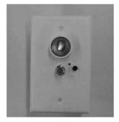
To use the TV antenna, turn "ON" the switch located on the TV jack. A red light will show on the indicating the antenna booster is powered. There will be a small continual 12-volt current drain as long as the switch is on. Turning the switch "OFF" changes the TV jack from antenna operation to park cable and ceases the current draw.
