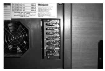
A 12-volt interior fuse panel is installed in the Power Distribution Center to protect the interior circuits. Circuit titles and fuse sizes are marked inside the access door. If a fuse blows, locate and correct the cause. Turn off all lights and motors, and then install a fuse with the same rating. If fuses continue to blow, a short circuit is indicated. Have the system checked by qualified personnel.
