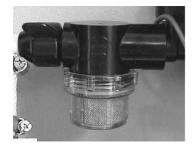
An in-line water filter attached to the inlet side of the water pump filters dirt, mineral scale, or organic matter out of the fresh water system. If you suspect a clogged filter, it is easily removed and cleaned. Loosen the clamp at the inlet end of the filter. Pull the water hose off the filter. Unscrew the filter from the water pump. Turn each end of the filter and pull apart.
