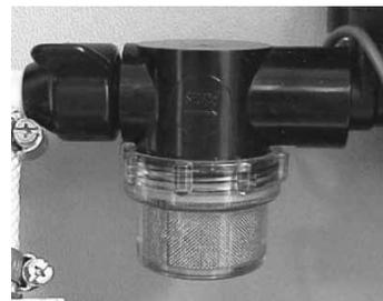
An in-line water filter attached to the inlet side of the water pump filters dirt, mineral scale, or organic matter out of the fresh water system. If you suspect a clogged filter, it is easily removed and cleaned. Loosen the clamp at the inlet end of the filter. Pull the water hose off the filter. Unscrew the filter from the water pump. Turn each end of the filter and pull apart.
