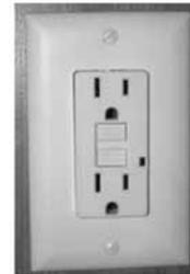
A Ground Fault Circuit Interrupter (GFCI) protects the bathroom, galley, and patio 120-volt receptacles. This device is intended to protect you against the hazards of line to ground electric faults and electrical leakage shocks possible when using appliances in damp areas.
