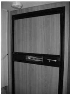
The refrigerator operates on 120-volt AC power or propane. The operating instructions supplied in the Owner's Information Package will help you with detailed information from the manufacturer.
